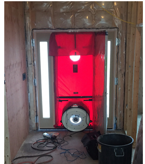
Image 3: An air tightness ("blower door") test during Mid-Construction Stage
