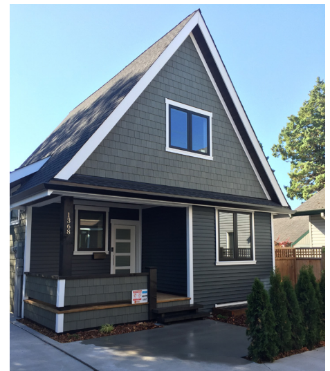
Image 2: The same Single Family Home (shown in Image 1) built to Step 4 of the Step Code shown after construction was completed.
