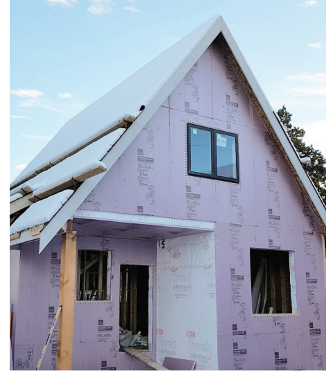
Image 1: A Single Detached Home designed to meet Step 4 of the Step Code, with exterior insulation shown during construction.
