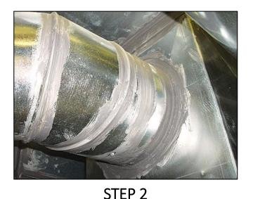
Duct sealing and visual inspection to confirm equipment installation meets design intent with appropriate standard of practice
