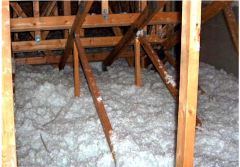
*Blown-in fibreglass attic insulation.*
