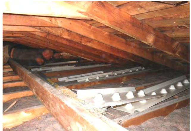
*Insulation baffles being installed at every second truss bay to provide opening from the soffit vents to the attic space, past the insulation (to be blown-in after).*
