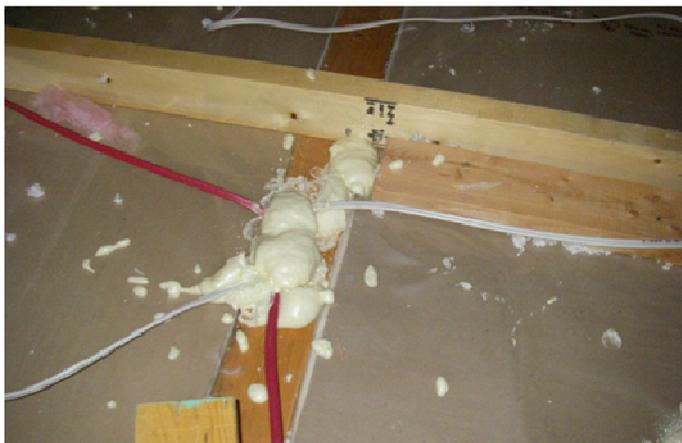
*Top plate penetrations sealed with sprayfoam.*
