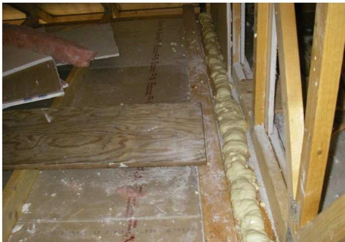
*Sprayfoam installed over top plate joint.*
