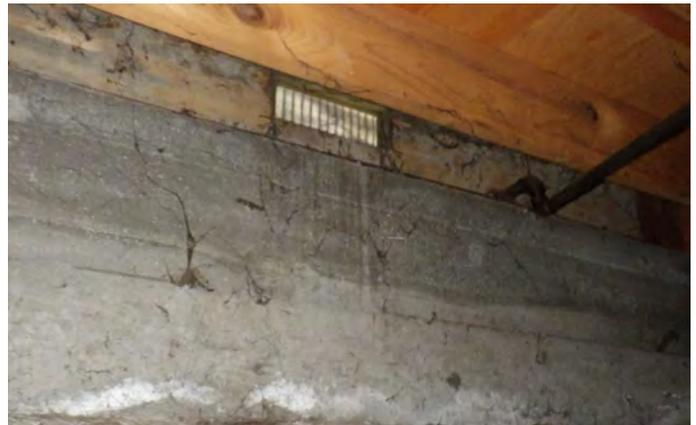
Air vent in the rim joist in an insulated vented crawlspace.
