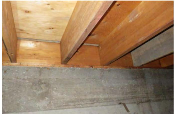
*Exposed below-grade wall at floor rim joist.*
