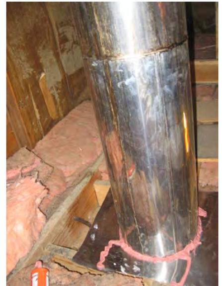
*Metal chimney with sheet metal seal over ceiling joists.*
